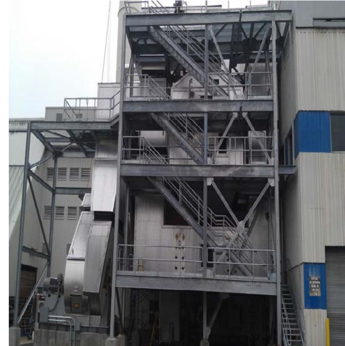
Vertical SCR with Bypass Duct and Reverse Flow Capabilities
