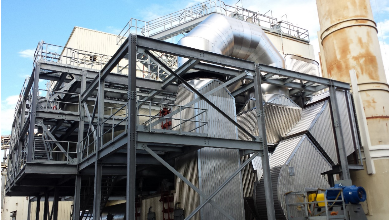
Horizontal SCR with Bypass Duct and Reverse Flow Capabilities
