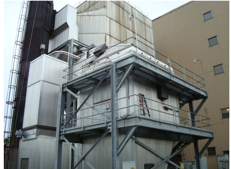
Vertical SCR with Bypass Duct and Reverse Flow Capabilities
