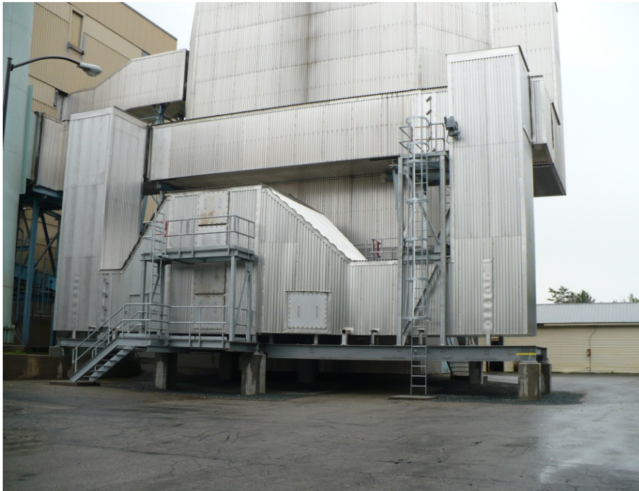
Horizontal SCR with Bypass Duct and Reverse Flow Capabilities
